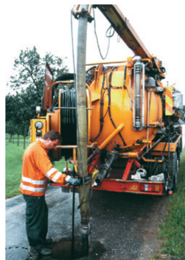
Nettoyage haute pression (ILLUSTRATION 19)
